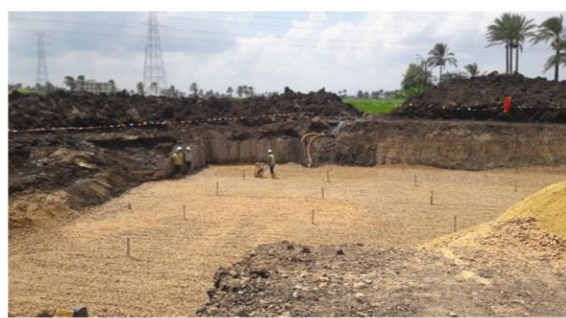
Soil replacement and compaction
