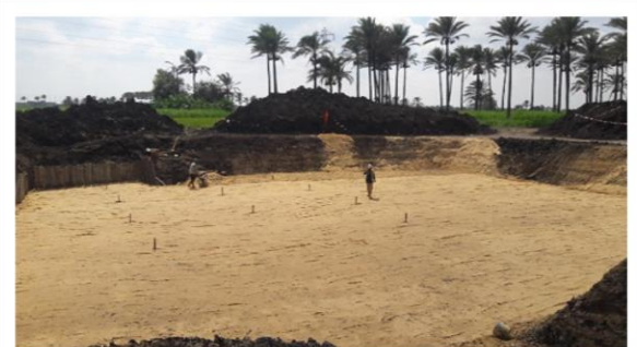
Soil replacement and compaction
