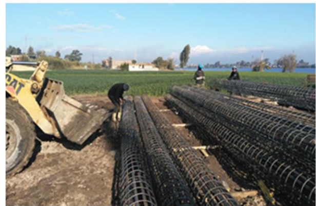
Deep Foundations (Piles) for OHTL
