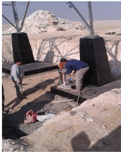
Core Test for Quality control
