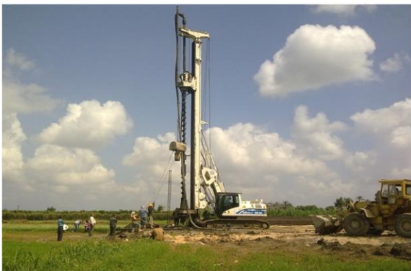
Deep Foundations (Piles) for OHTL
