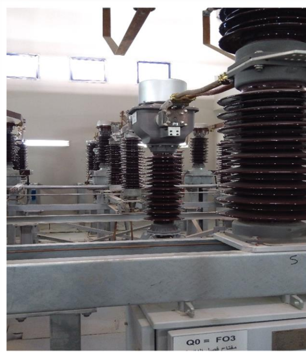
Conventional Indoor 66 kV Equipment
