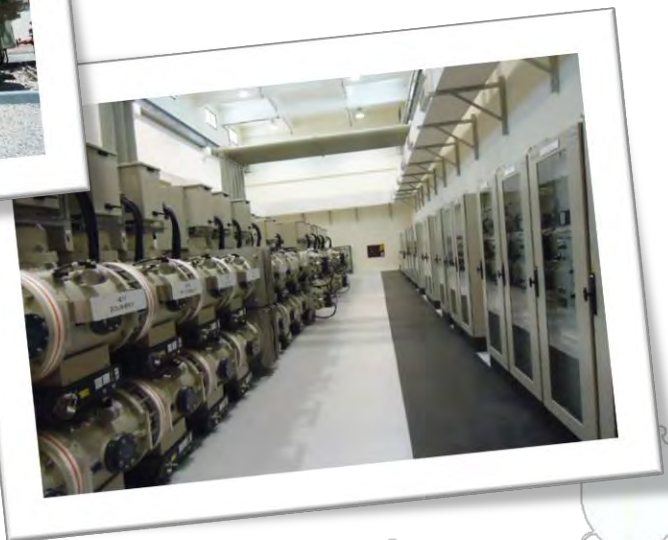
Main AC/DC Relay Sub AC/DC
