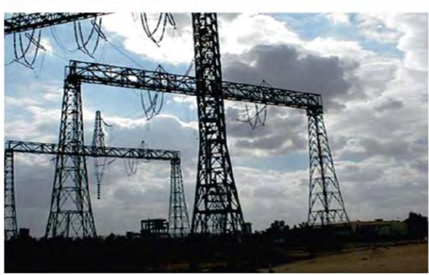
High Voltage testing station Repair of Steel Structure & Foundation
