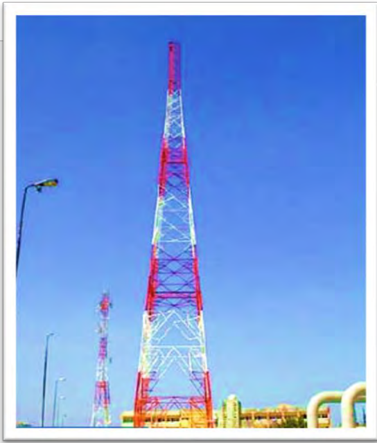
Design & Construction Supervision Of MicroWave Towers
