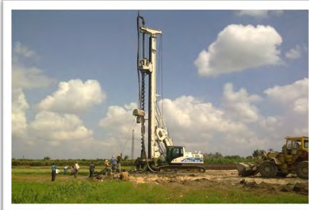
Deep Foundations (Piles) for OHTL
