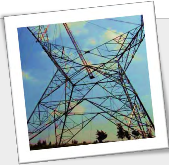
500 kV Single Circuit Tower
