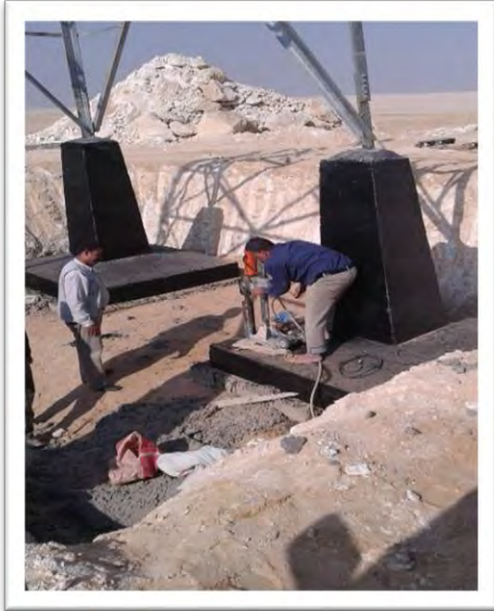
Core Test for Quality control
