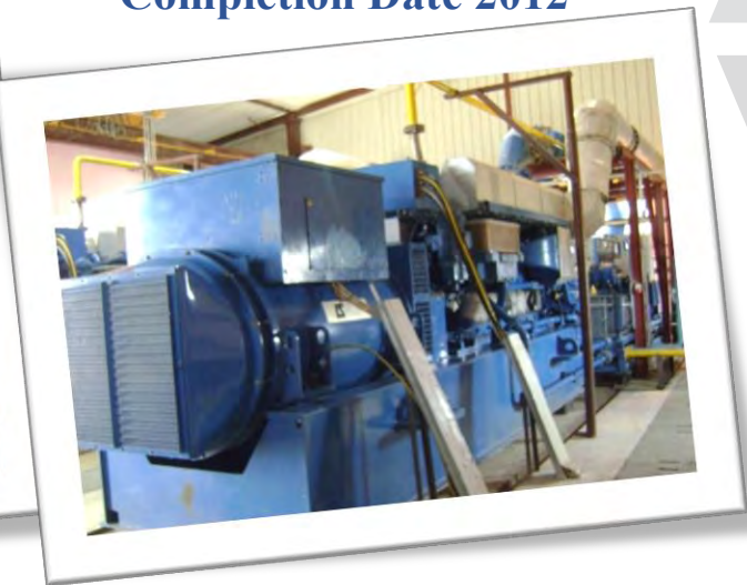
Diesel engines inside engine hall
