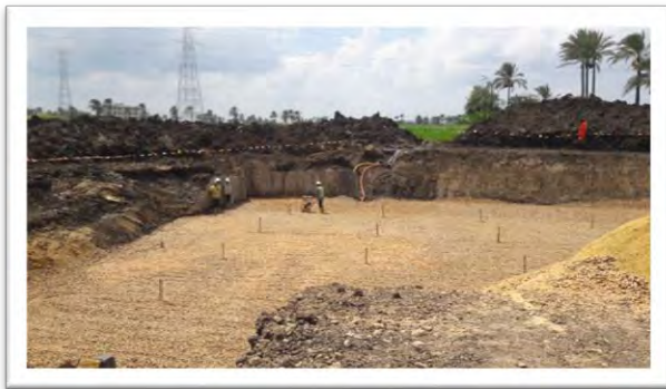
Soil replacement and compaction
