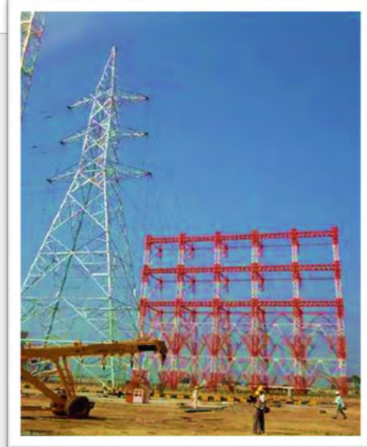
Loading test for Towers
