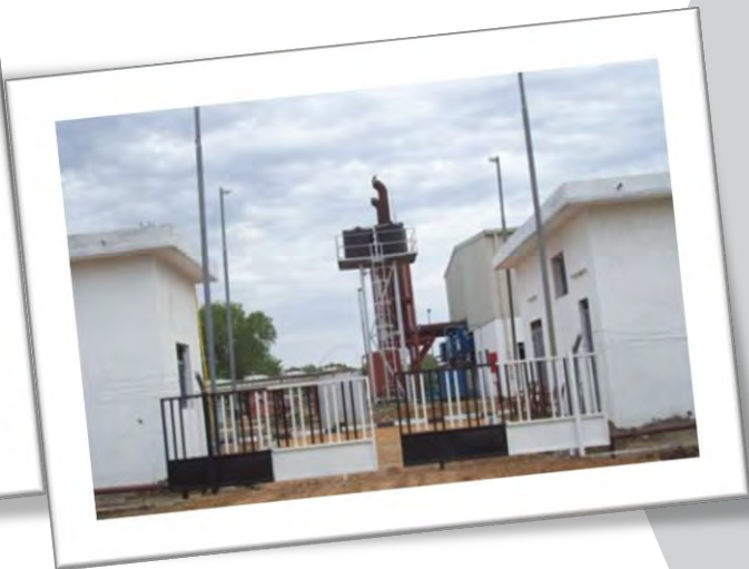
Bor Power Plant Main Entrance
