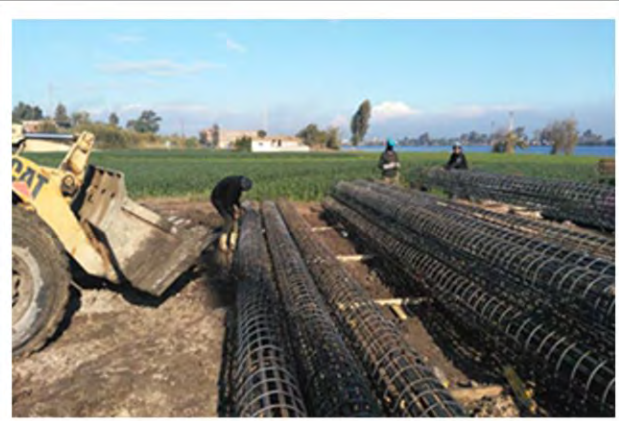
Deep Foundations (Piles) for OHTL
