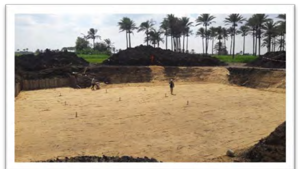
Soil replacement and compaction
