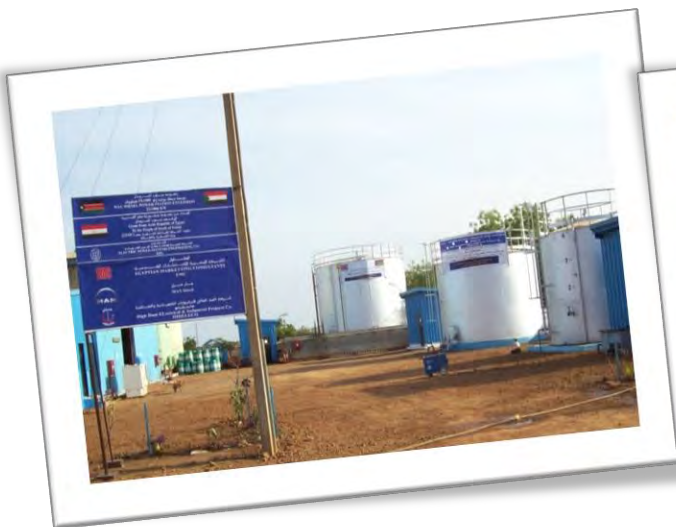
Wau Power plant over View
