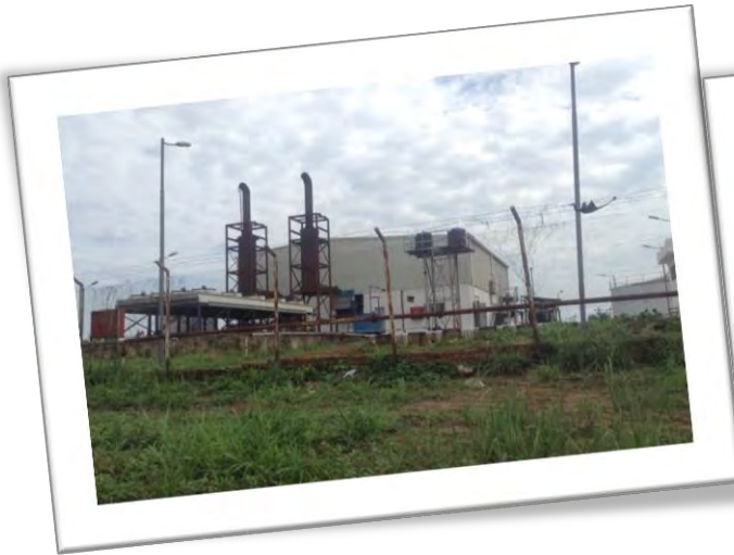
Yambio Power plant over View
