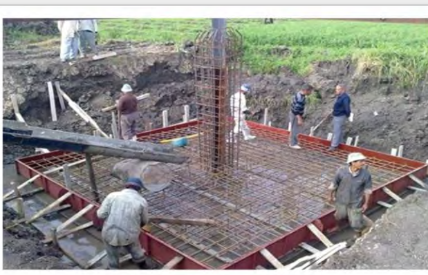
Foundation for OHTL
