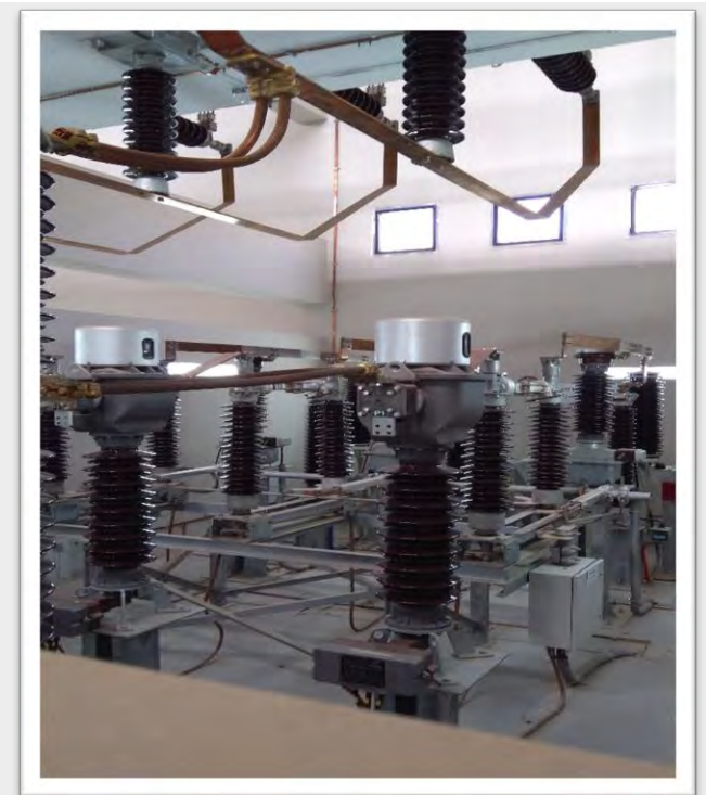
Conventional Indoor 66 kV Equipment
