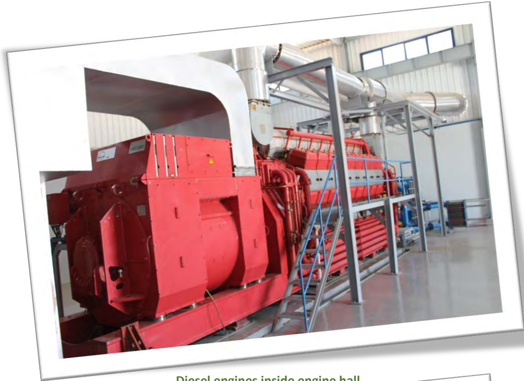
Diesel engines inside engine hall
