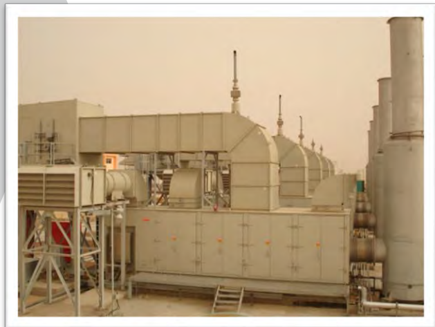
Karama Power Plant
