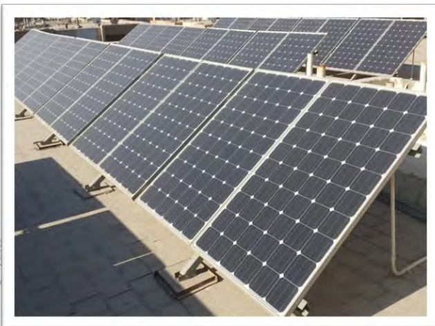
PV Solar power stations
