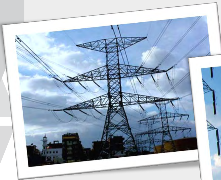
500 kV Double Circuit Tower
