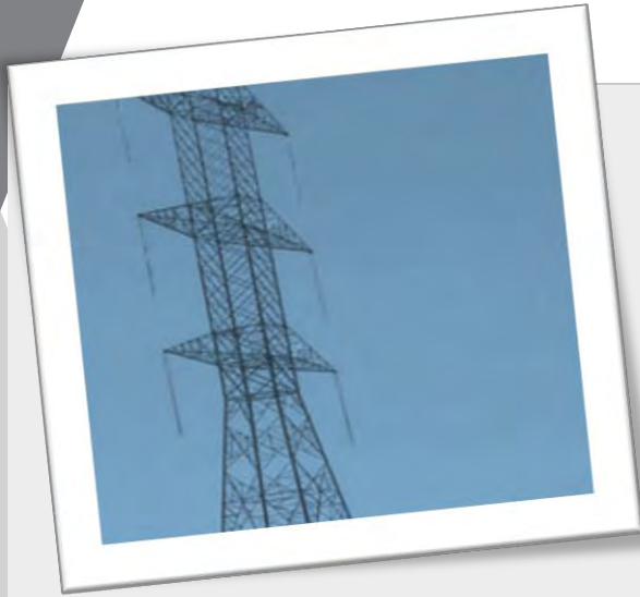
500 kV Double Circuit Tower
