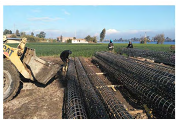
Deep Foundations (Piles) for OHTL
