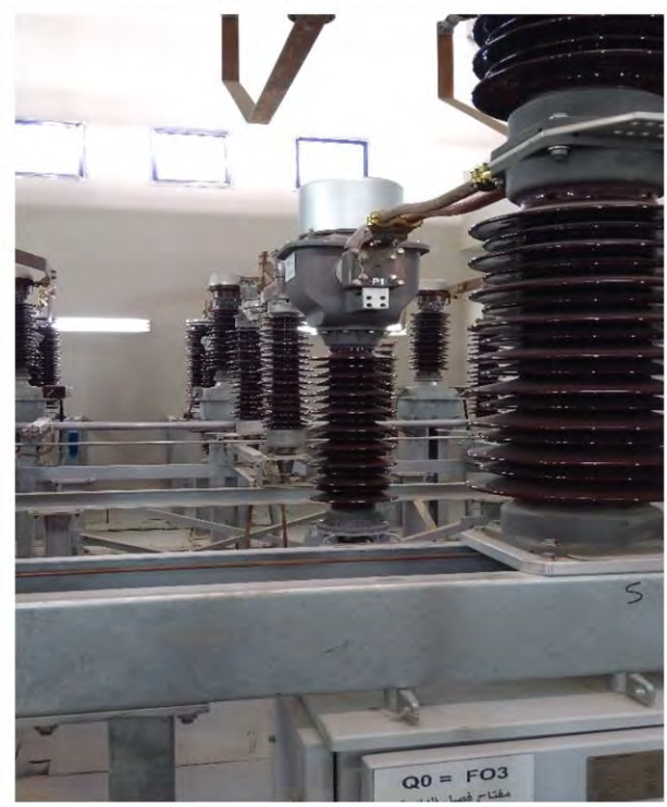
Conventional Indoor 66 kV Equipment
