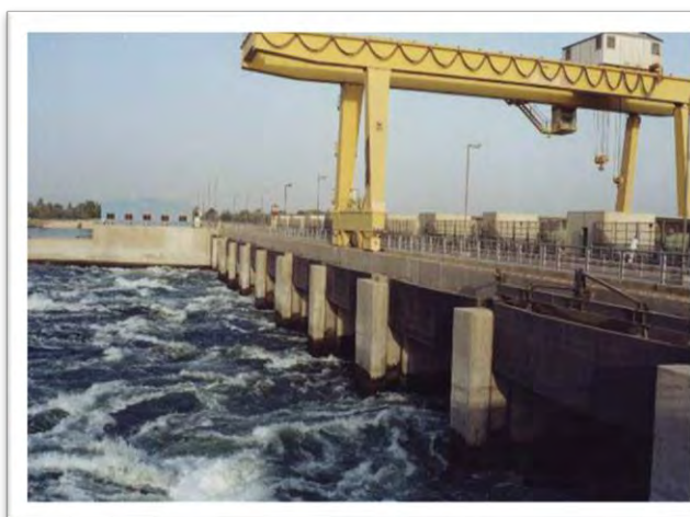
ESNA Hydro Power Plant
