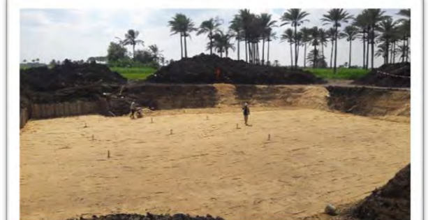
Soil replacement and compaction
