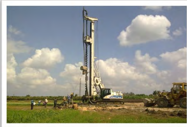
Deep Foundations (Piles) for OHTL
