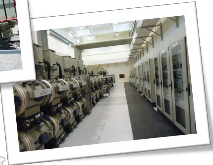
New Ghobrah 132/33/11 KV GIS S/St
