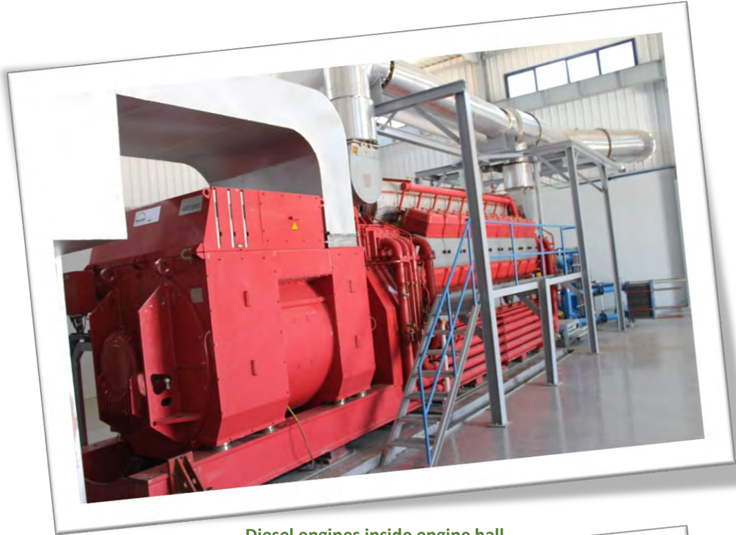
Diesel engines inside engine hall
