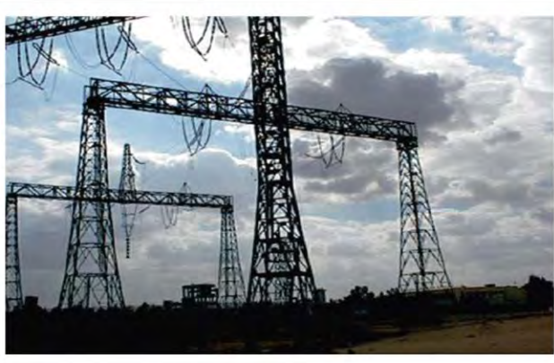
High Voltage testing station Repair of Steel Structure & Foundation
