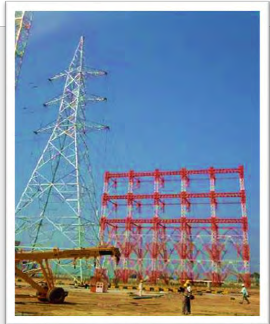
Loading test for Towers
