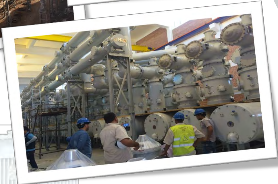
Suez Gulf 500/220 KV GIS Substation 1x500 MVA
