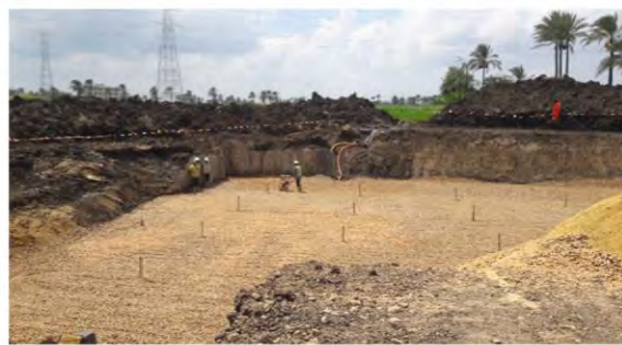
Soil replacement and compaction
