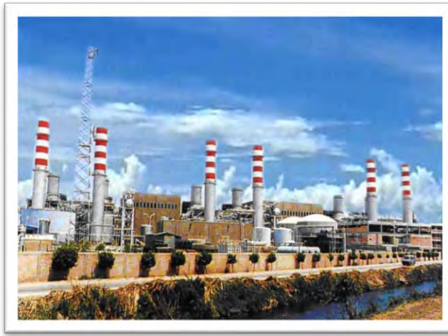
Damietta Combined Cycle Power Station
