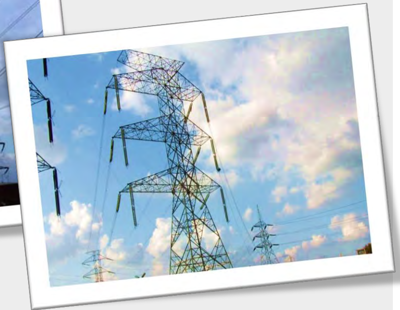
Multi Circuits Towers Approach to El-Siouf Substation
