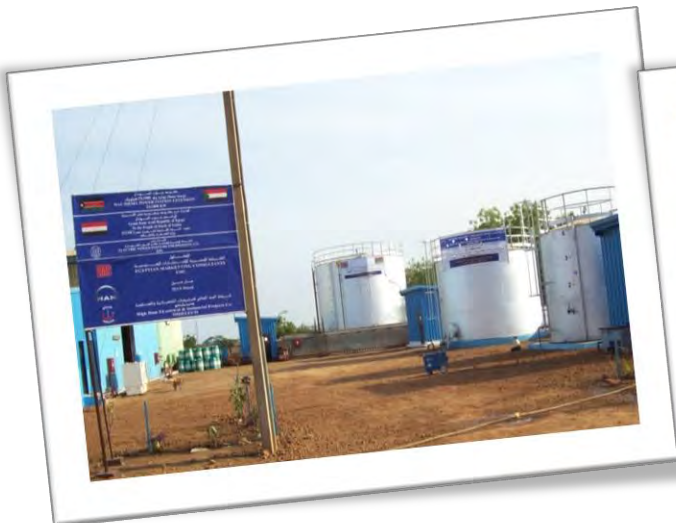
Wau Power plant over View
