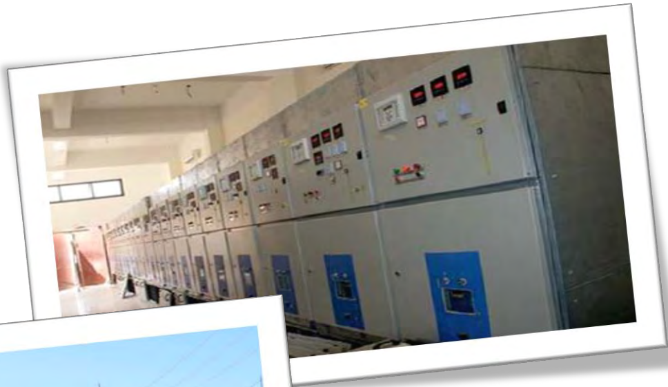
Medium voltage Switchgear
