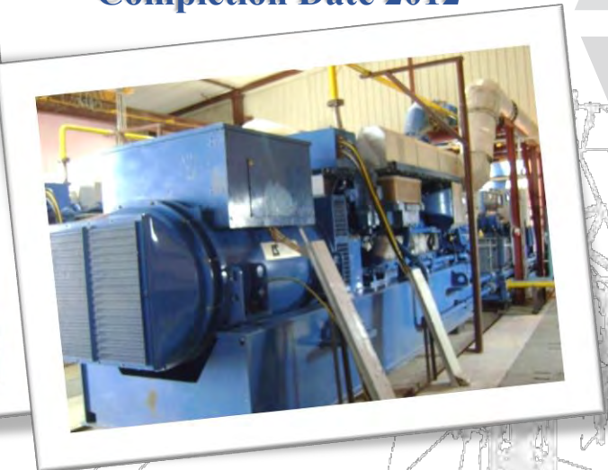
Diesel engines inside engine hall
