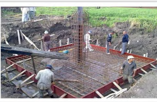
Foundation for OHTL
